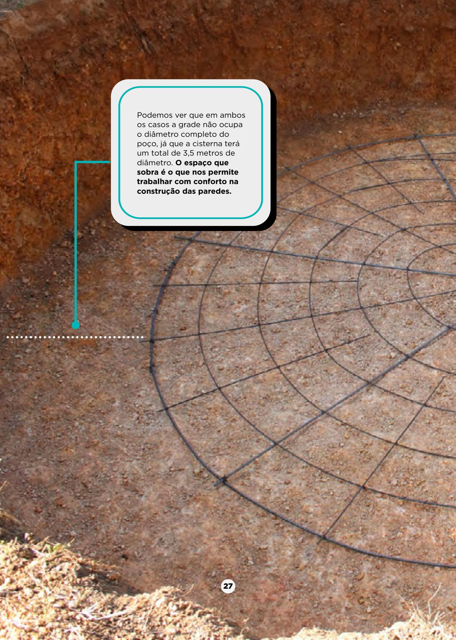
A photograph of a circular well under construction. The floor of the well is covered with a grid of black rebar. The walls are made of reddish-brown earth. A white callout box with a teal border is positioned in the upper left quadrant, containing text. A teal line connects the box to the rebar grid. A dotted white line extends horizontally from the end of the teal line.
